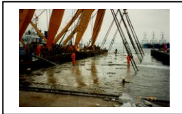
Concrete Pontoon, Rostock
