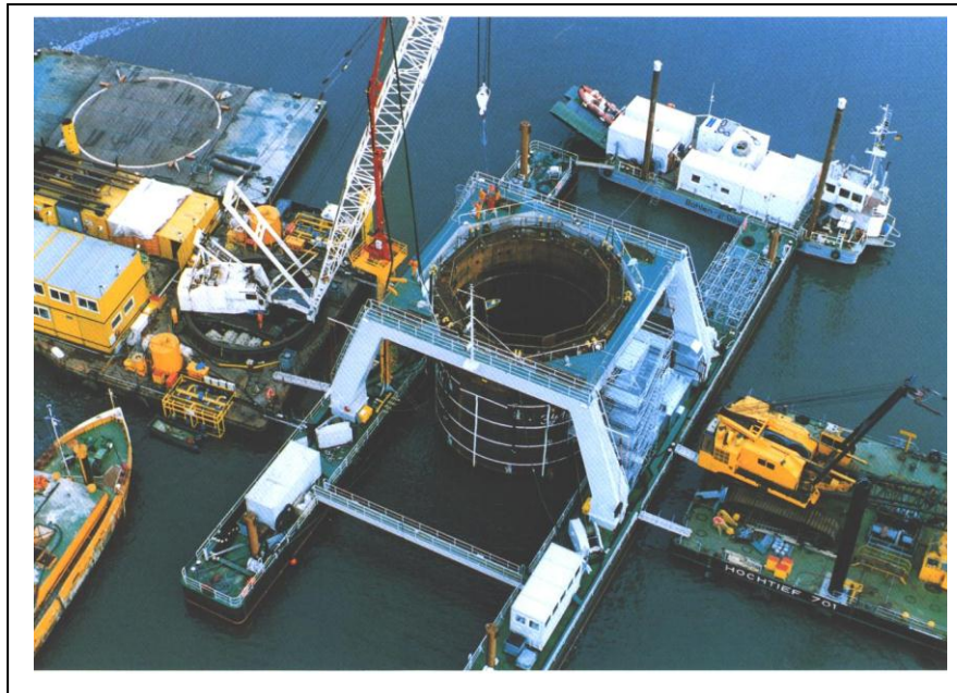
Tie In Chamber Europipe I and II, Germany
