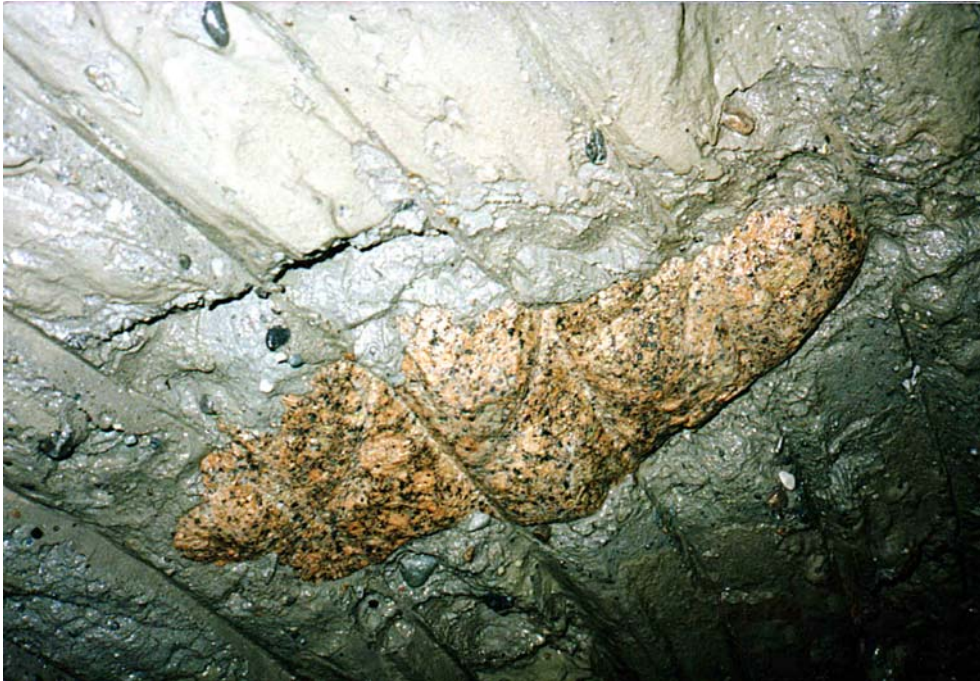
Figure 16: Boulder ground down
