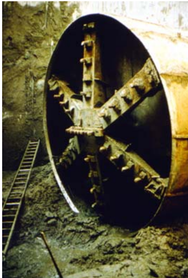
Figure 13: Prototype Slurry TBM 1974
